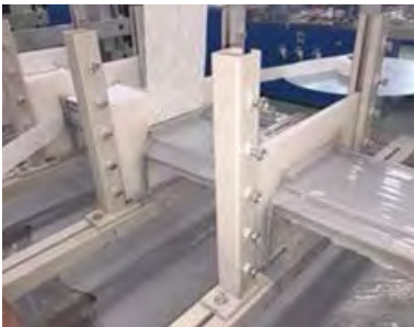
Standard Cable Ladder and Cable Tray fittings are fabricated using SS angle plates and SS bolt sets unless stated otherwise.
